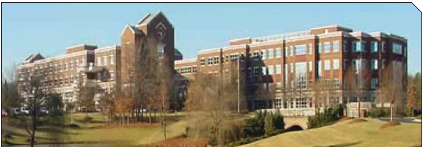
FIGURE 6. A hospital in the Southeast employed a BAS design for control and energy savings.
